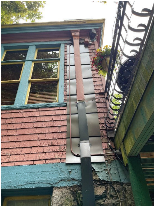
Figure 3: Gutter and Down Spout
