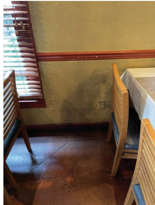
Figure 4: Main Level Interior Wall Patch
